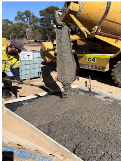
Photo 1: Pouring of Collicrete
